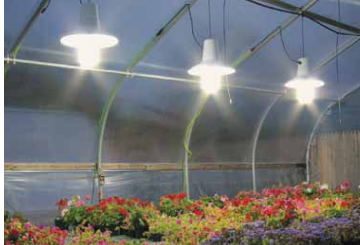
Reflectors enhance light emission and increase coverage area, reducing the number of required fixtures.
