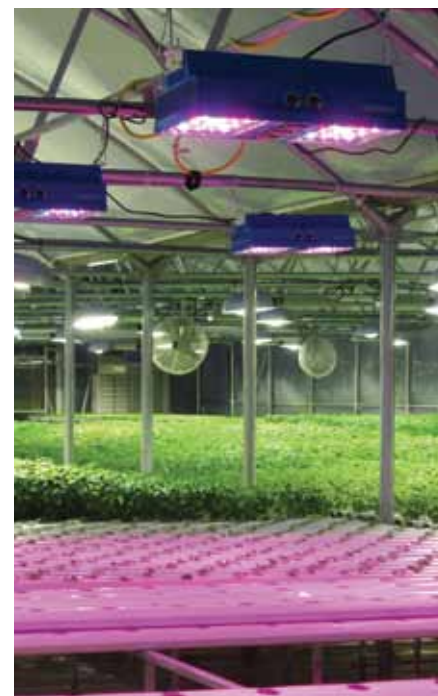
LEDs are highly efficient and have low energy requirements. Some LEDs are rated for up to 50,000 light hours.
