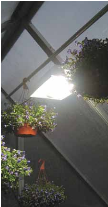
Full spectrum compact fluorescent lighting closely resembles actual sunlight and provides a balance between cool and warm light.
